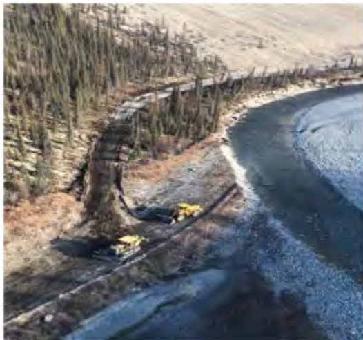
Connection of road at KP 4
