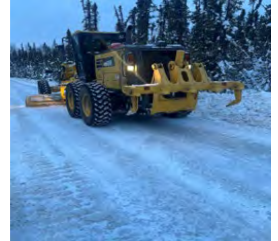
Grader on road making touch ups at KP158
